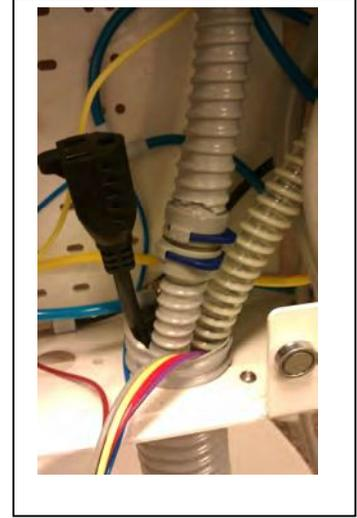
17. Remove the cap from the large water supply line, Connect the water supply line to the cuspidor. Remove the cap from the signal air line, then connect it to the cuspidor.
