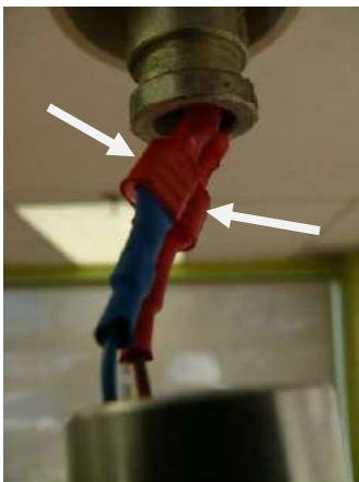
Figure 73: Connect the 2 wires from the lamp head to the 2 wires from the arm. It does not matter which wire is connected to which wire.
