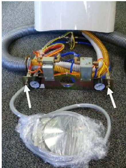
Figure 84: Install the utility box. This should be placed on the floor where the air, water and suction lines are located.
