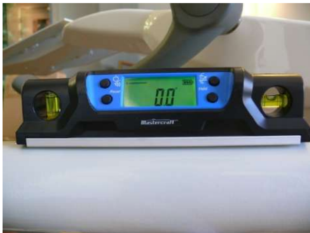
Figure 13: Place a level on the bracket and adjust the jacking setscrews and bolts as needed to get a perfect level.
