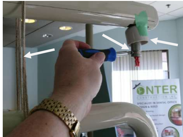
Figure 72: Install the big plastic cover at the top of the arm. Use tape to hold it up. Use rope to hold the arm down. Remove the screw at the end of the arm.
