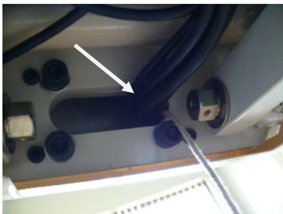
Figure 11: The cables will be passed through this oval opening. Pass the cables through and let them out from the bottom of the post hole.
